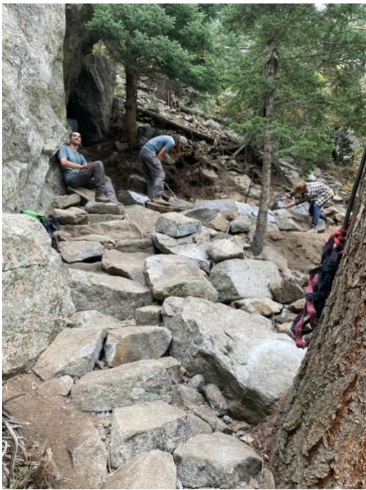
Figure 2: Stone structures were built to facilitate the trail and prevent erosion of the hillside.
