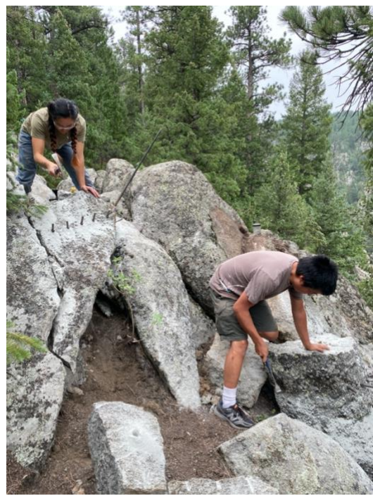
Figure 3: Volunteers learning to quarry and split stone.
