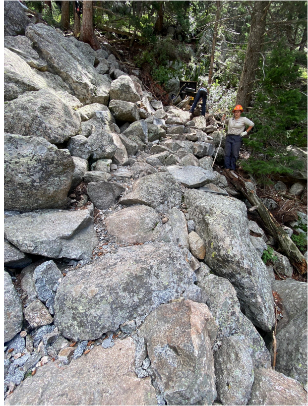
Figure 5&6: Tread created through the upper talus field via shifting large rocks to a stable position. (Phase III)
