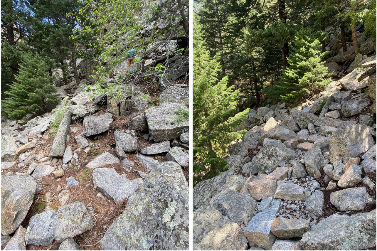
Figure 3&4: Stone steps and tread with retaining structure heading up through some more stable talus. (Phase III)
