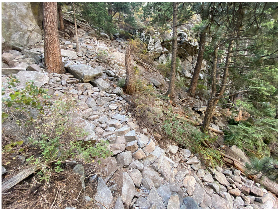
Figure 9 & 10: Staircase with retaining structure heading to Middle wall. (Phase I)
