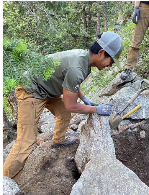
Figure 2: BCC trails staff setting a rock
