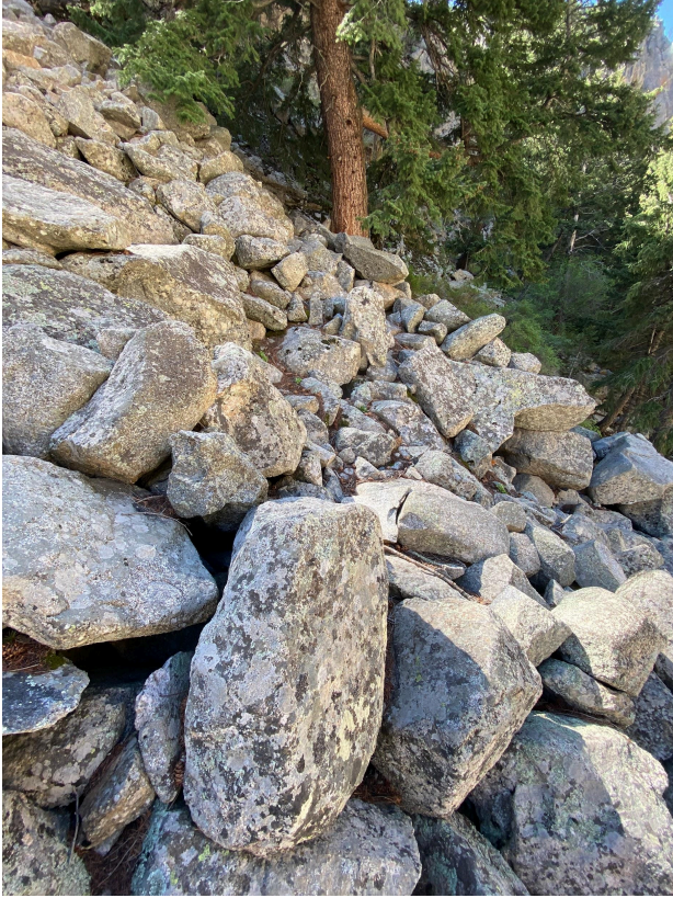
Figure 5&6: Tread created through the upper talus field via shifting large rocks to a stable position. (Phase III)
