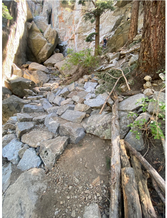
Figure 11 & 12: Heavily eroded trail up to the main wall at Avalon. A large retaining wall with the trail running through it was built to stabilize the trail and hillside while diverting the main trail to a more stable surface. (Phase II)
