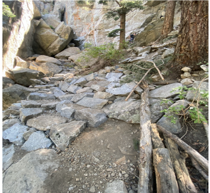
Figure 1: Trail reroute to more durable surfaces
