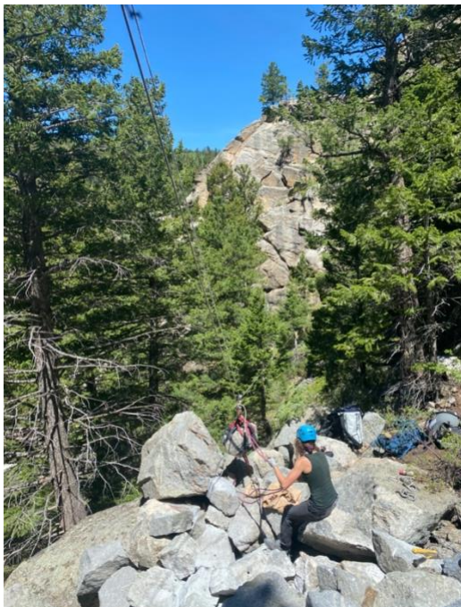
Figure 4- FRCS staff utilizing the highline system to transport material
