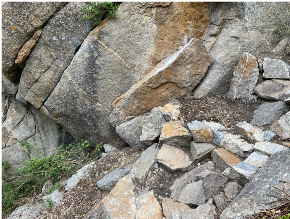
Figure 3- Construction of a belay pad, providing a sustainable and flat area to stage and climb from.
