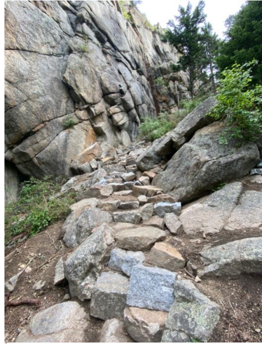
After: Access to climbs at Broken Rock
