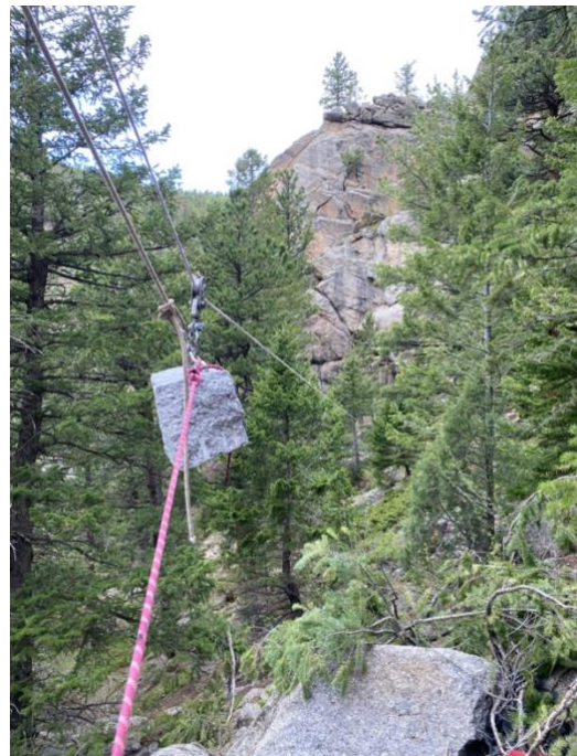
Figure 5- Material being transported via the highline.
