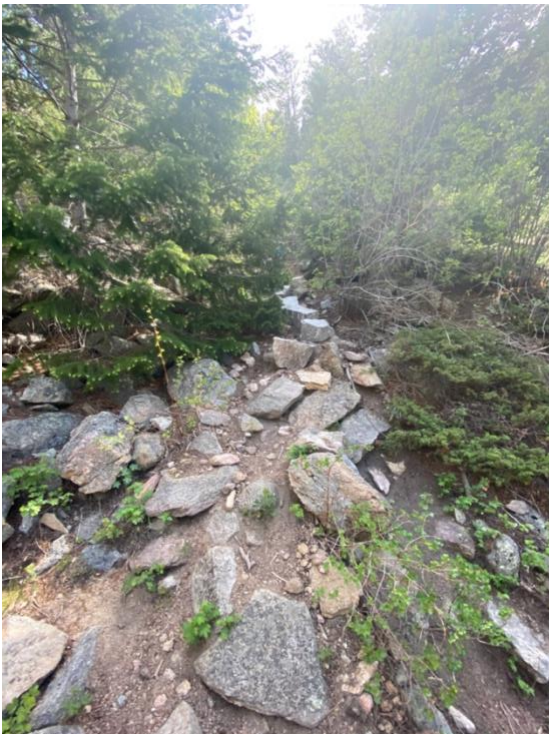
Before: Erosion on the primary user trail
