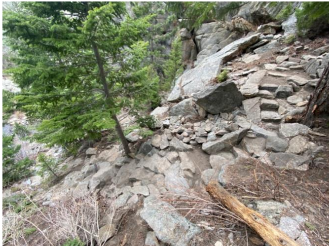
Figure 1- Construction of a primary path out of durable stone material
