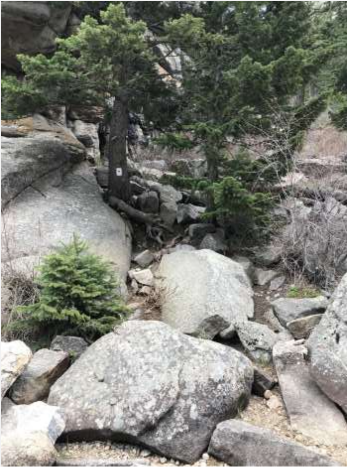
Figure 4 - Eroded slope above creek bed (Before)
