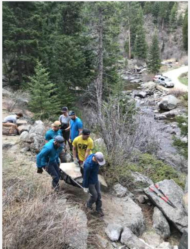
Figure 3 - Volunteers from Rab transporting the stone material
