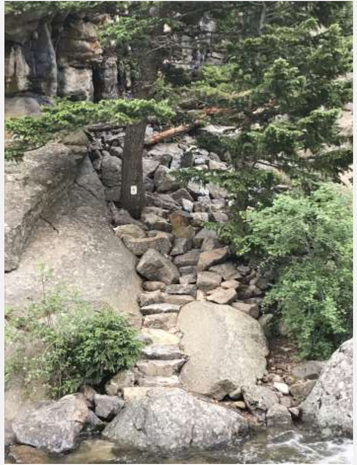
Figure 4 - Erratic, yet functional steps/structure at start of trail (After)
