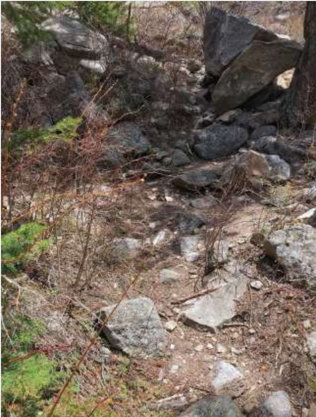
Eroded Trail; Section A - Before
