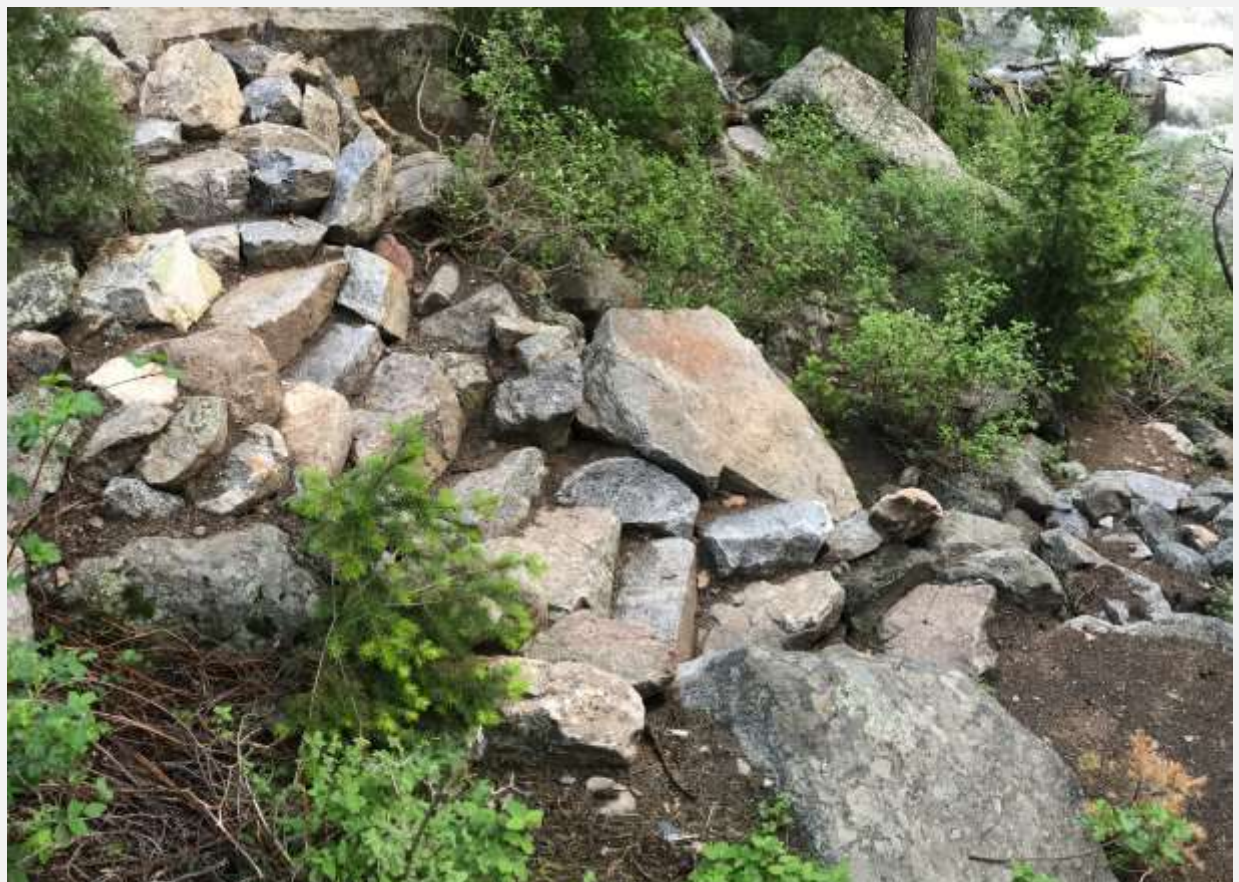
Restored Trail; Section C - After
