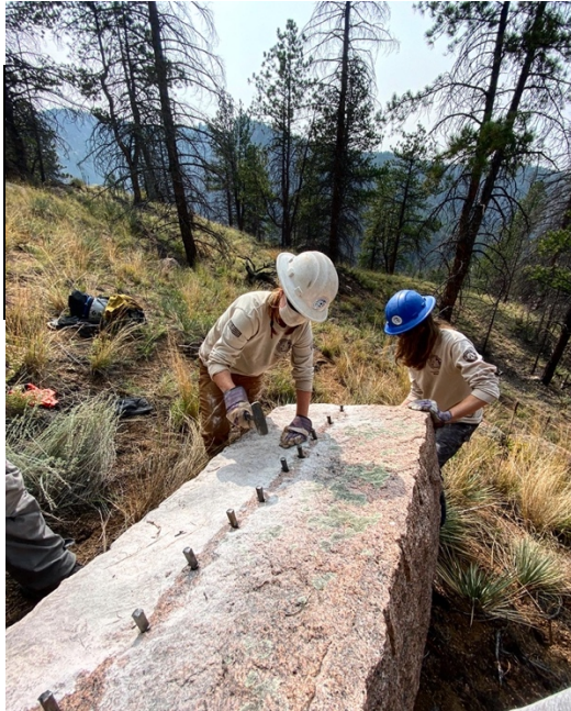
Figure 2: ACE crew members learning to split stone using feathers and wedges.
