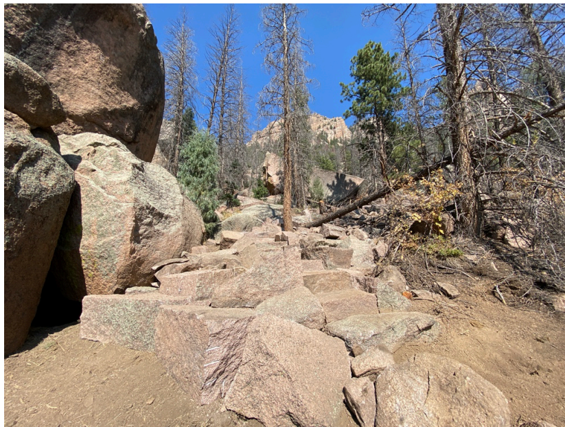
Figure14: Stone steps built through upper quarry at the location of Figure 13 After (2020)
