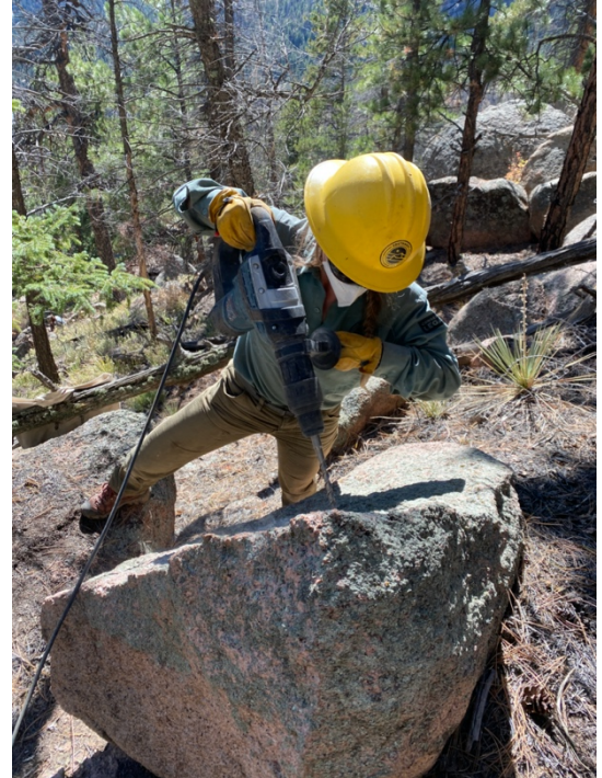
Figure 6: SWCC crew member quarrying a rock for a stone structure (2021)
