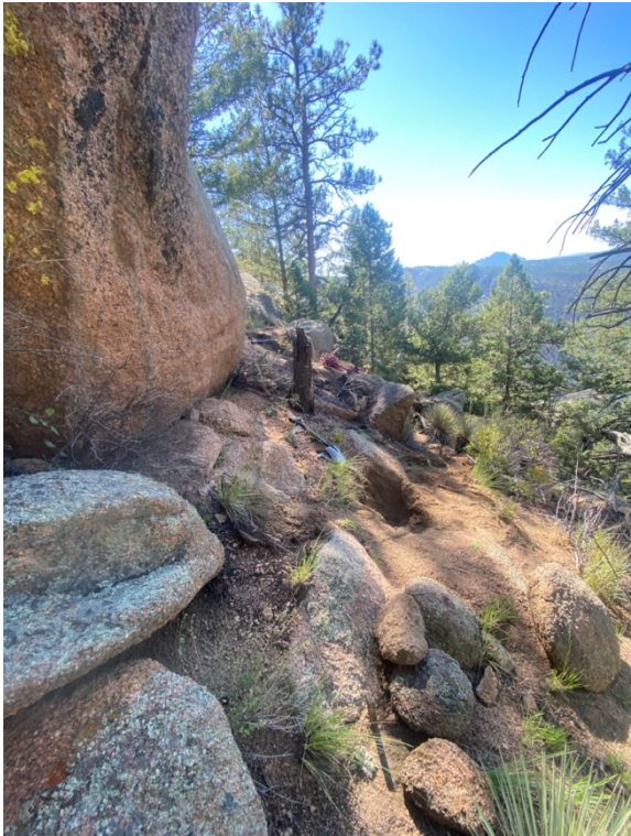
Figure 25: Rocky uneven surfaces where new tread will be constructed Before (2022)
