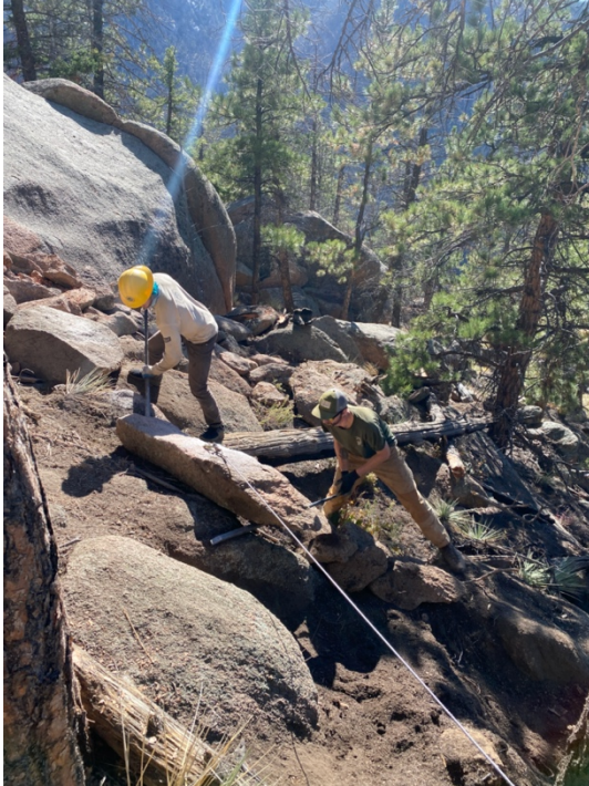
Figure 5: BCC and SWCC crew rigging and moving a rock into place (2021)
