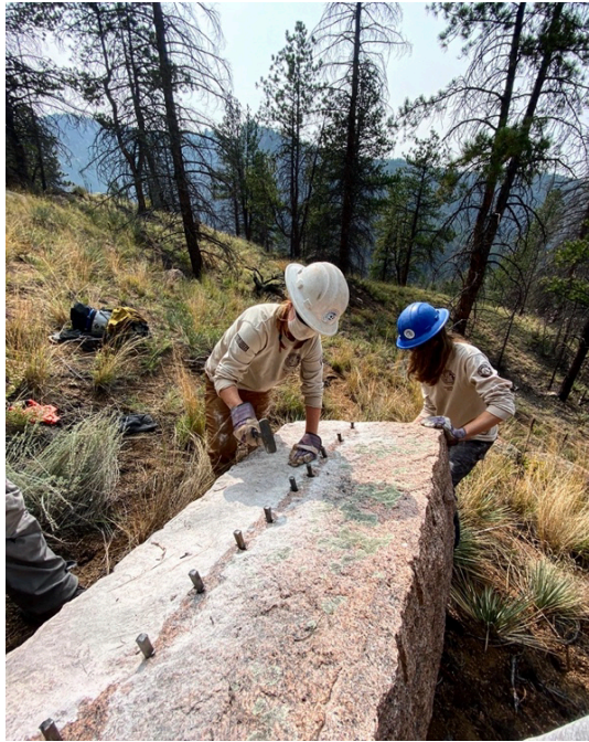
Figure 2: Ace crew members learning to split stone using feathers and wedges (2020)
