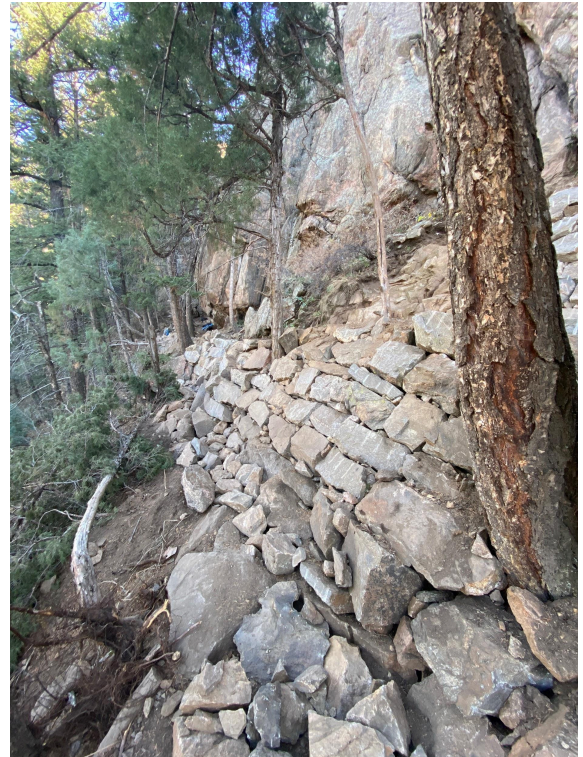
Figure 1: 20 ft long retaining wall
