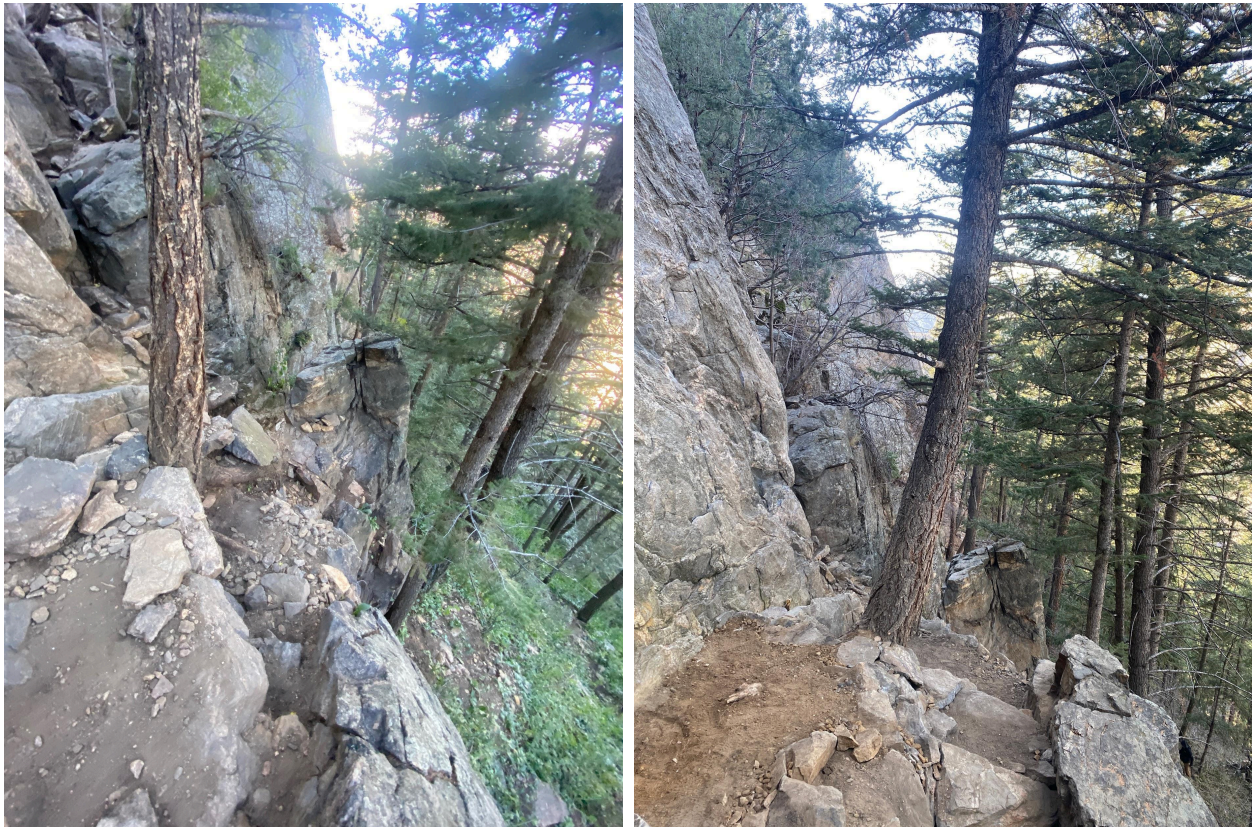
Figures 14 and 15: The base of the eroding East Wall (left) is now built up with a stone retaining structure and now has a large belay pad for the three climbing routes (right).
