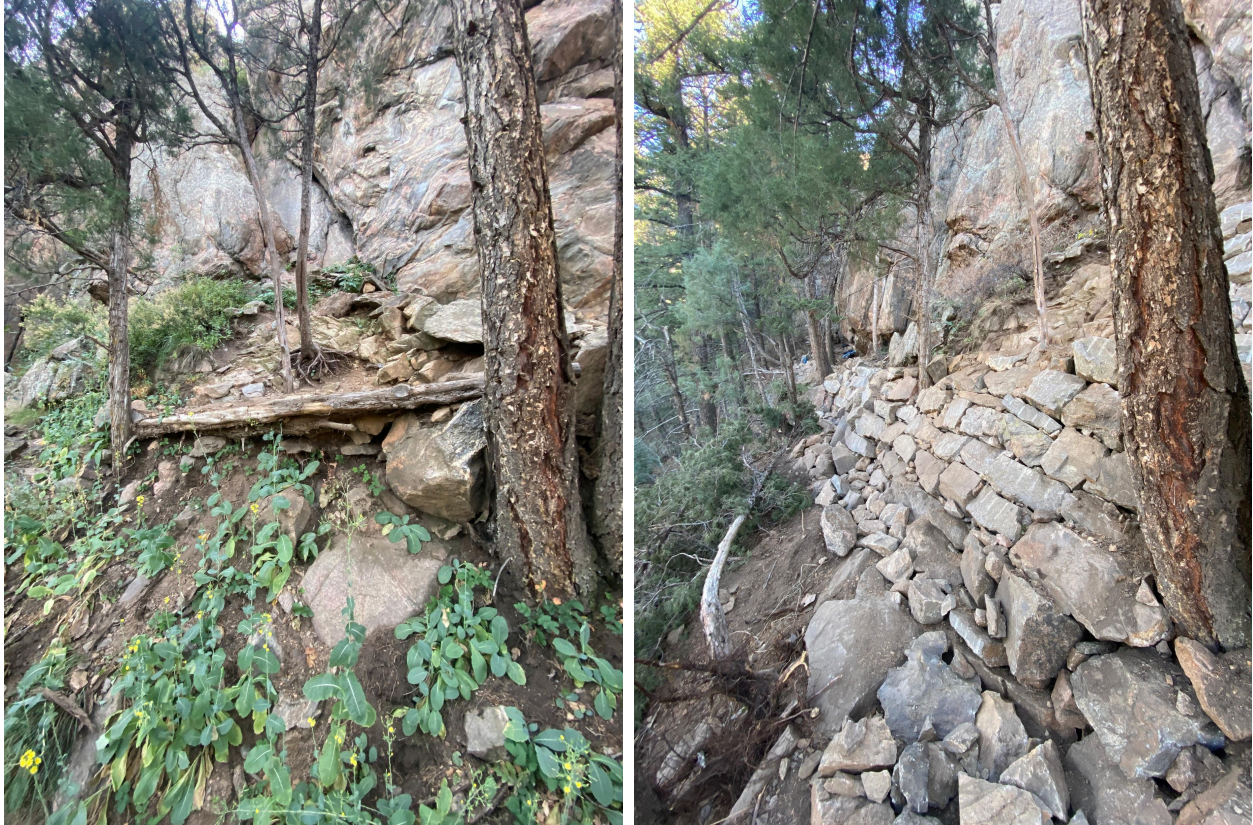
Figures 6 and 7: Old trail held up by a singular dead log (left) replaced with a large stone retaining wall (right).
