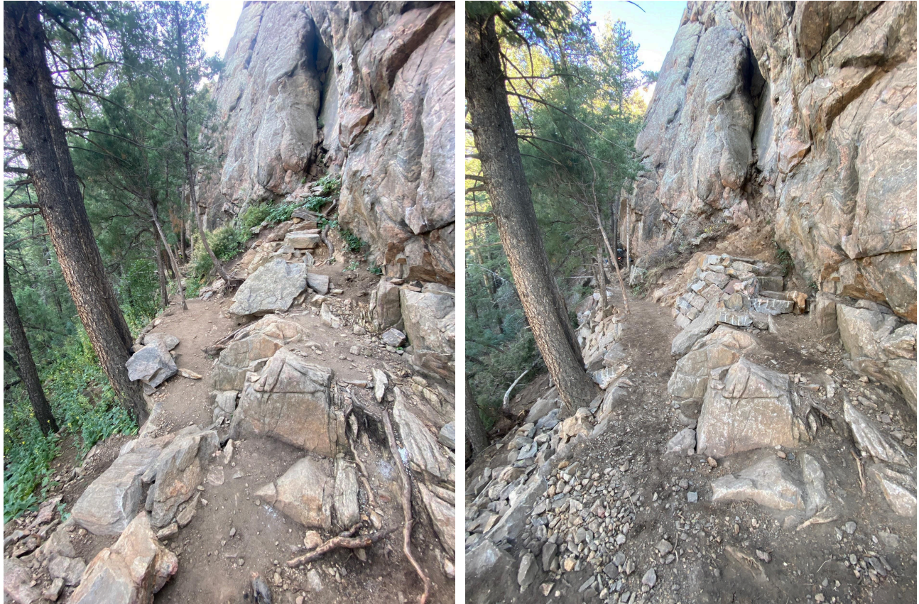
Figures 4 and 5: Eroding trail and loose belay pad (left) turned into a durable trail supported by a stone retaining wall and a sustainable stone belay pad for Three Little Birds 5.9 (right).
