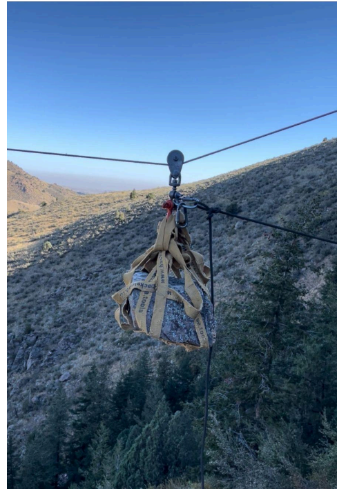
Figure 2: Rock loaded up in the BCC's highline rigging system.
