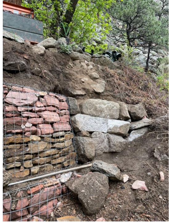
Figure 3: Gabion baskets flowing into a traditional stone structure
