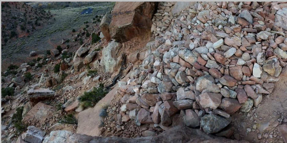
After – Retained slope with hardened surface that detracts use
