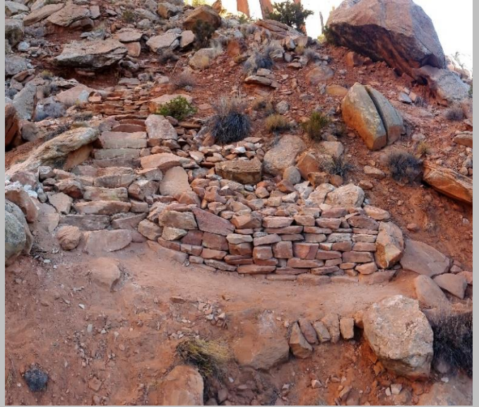
After – rebuilt and enhanced structures
