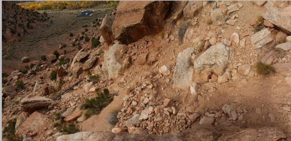
Before – eroded slope that appears like trail
