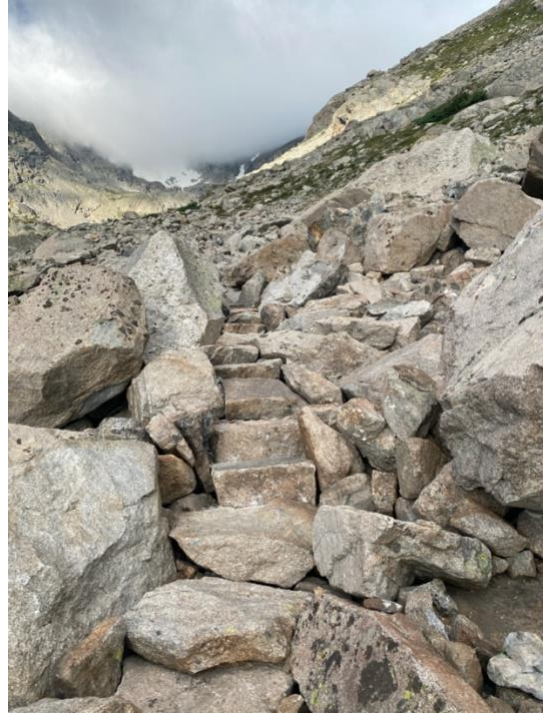
Figure 3: Stone staircase constructed without shaping or manufacturing stone.
