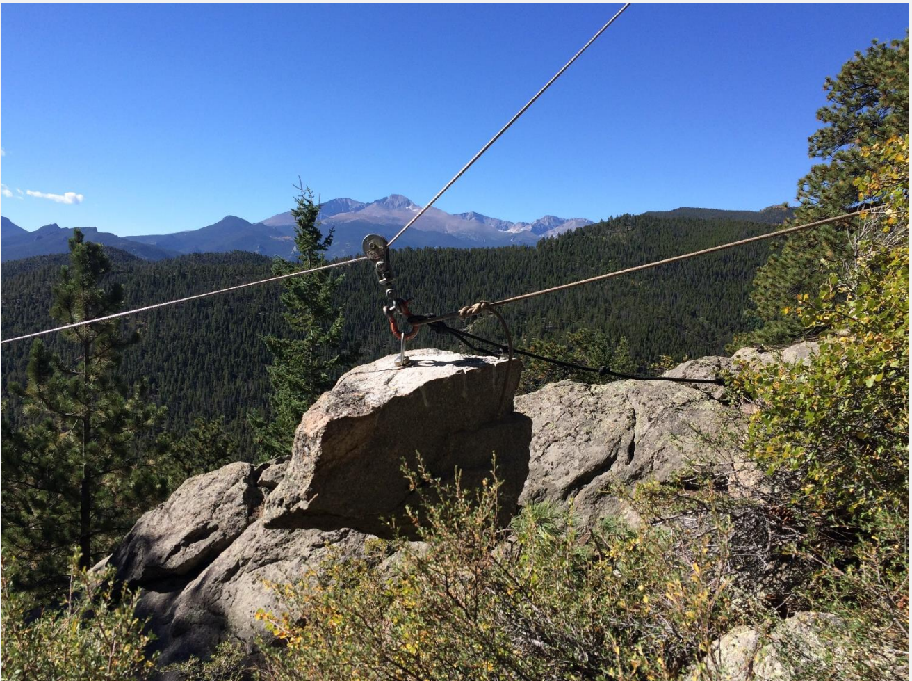
Figure 5 – Highline transport of materials
