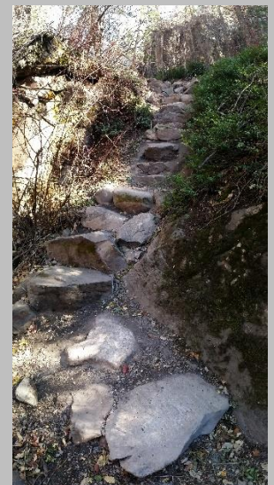
After – hardened staircase
