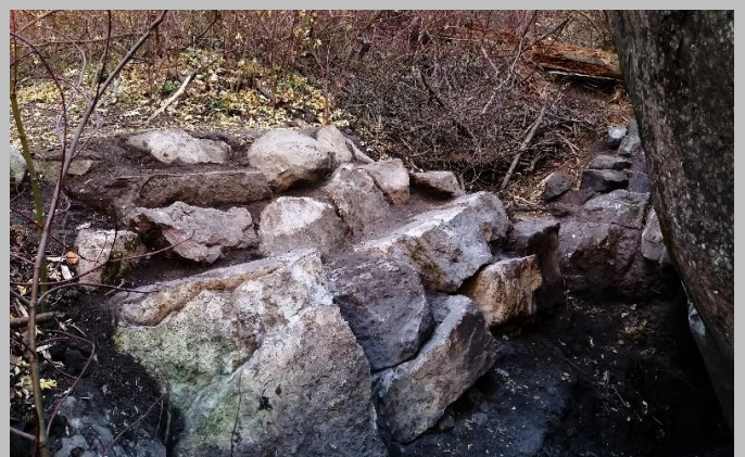
After – hardened trail tread & drain
