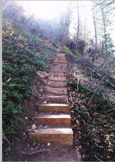
After – Timber risers
