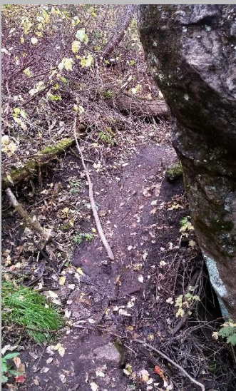
Before – eroded slick slope
