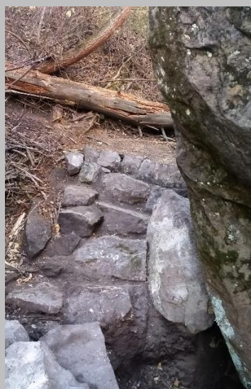
After – hardened staircase
