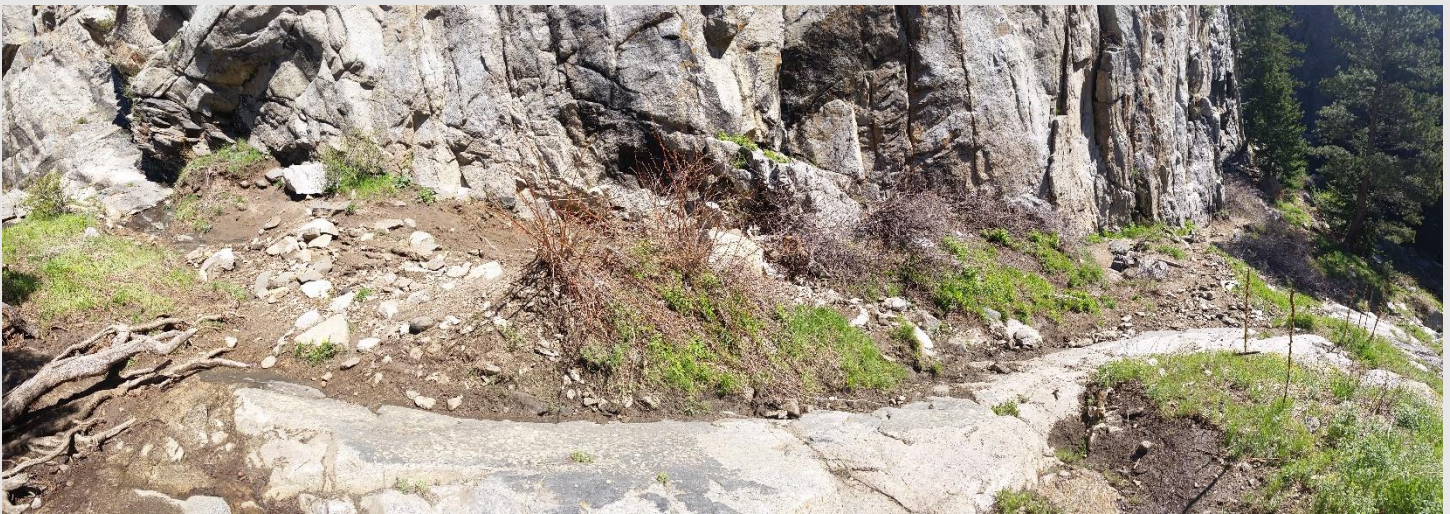
Figure 1 - Erosive slope before
