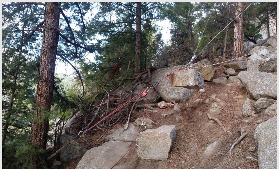
Figure 2 - Rigging Rock material into position
