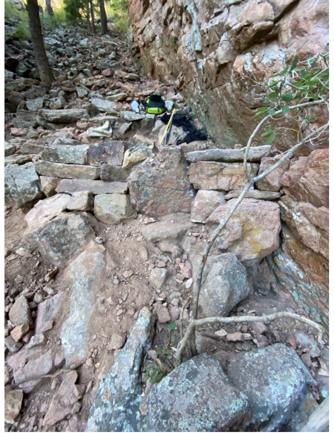
Figure 13: Retaining structure for the belay pad incorporating existing solid stone. After
