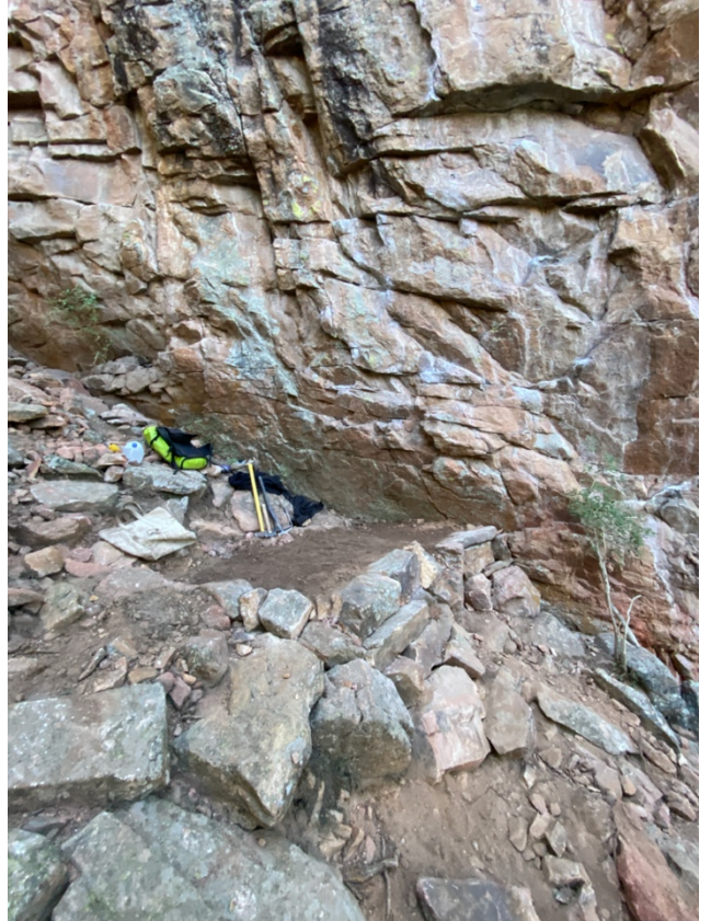
Figure 11: Belay pad constructed with retaining structure. After
