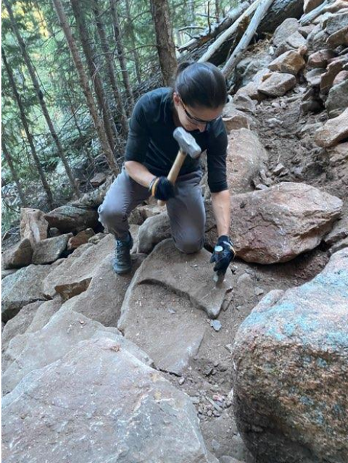
Figure 1: Volunteer shaping a rock with a chisel
