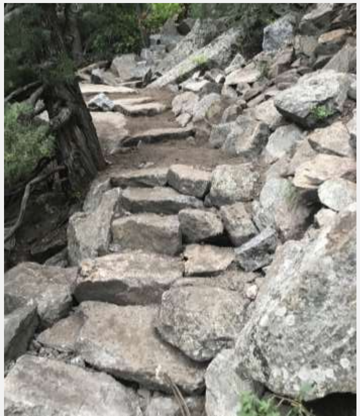
Figure 6 - New tread alignment (after)
