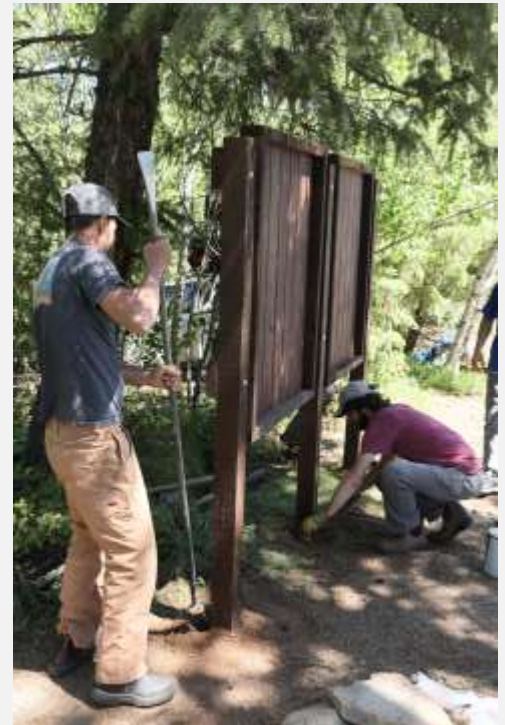
Figure 4 - Installing informational kiosk
