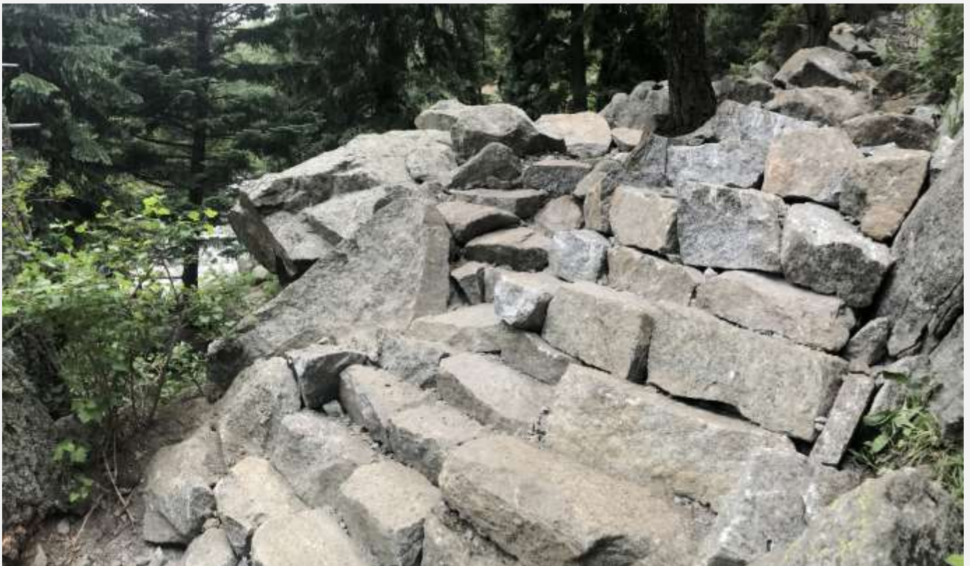
Figure 7 - Retaining structure near S Boulder Creek
