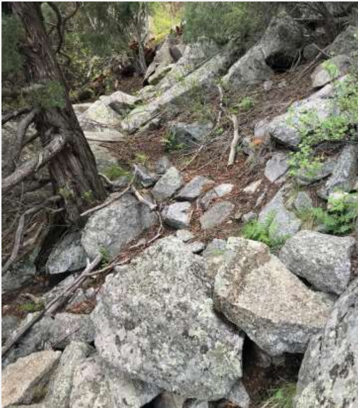
Figure 6 - New tread alignment (before)
