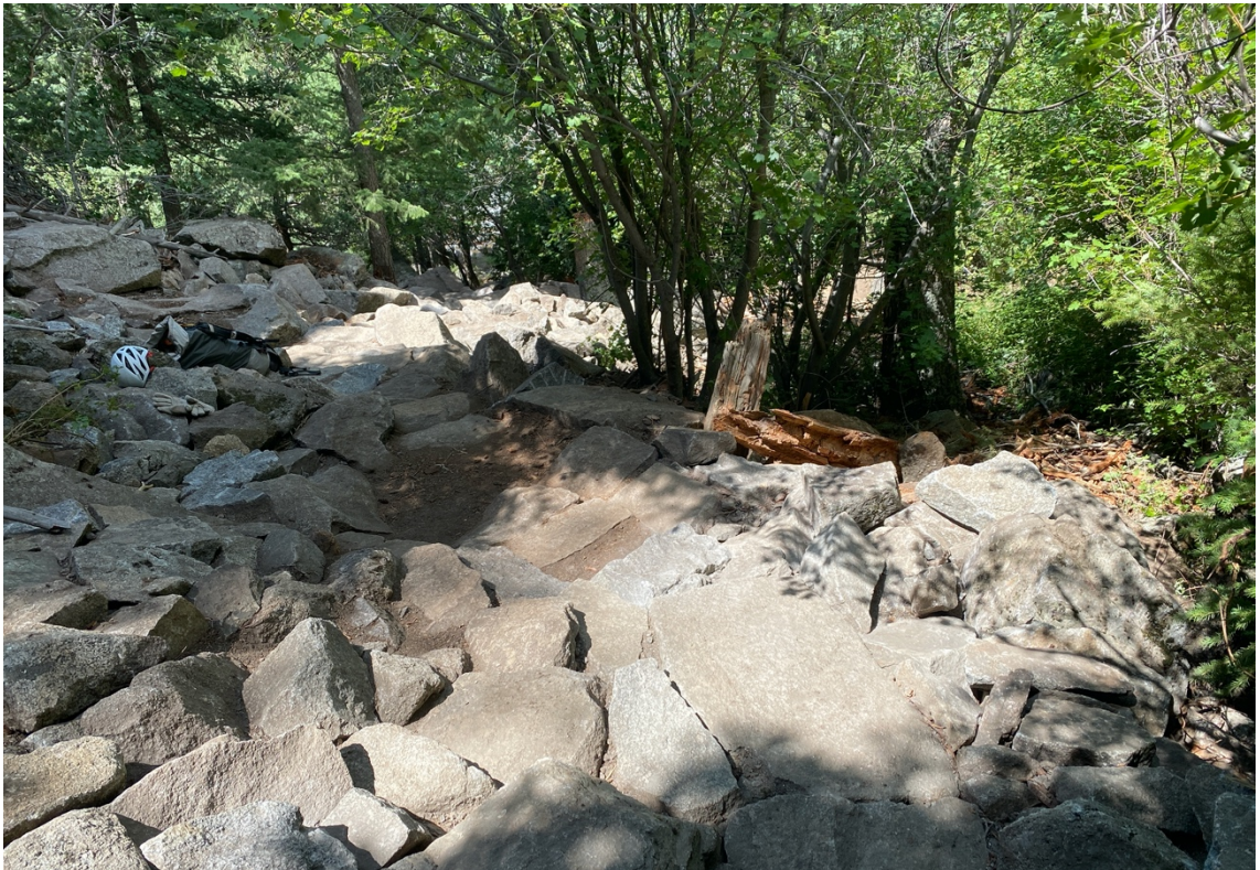
After: The original trail was decommissioned and restored and a sustainable path was built through the adjacent talus field.
