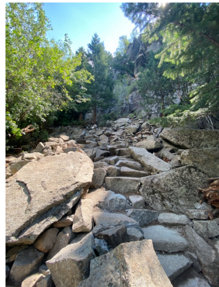
Figure 1: FRCS moved the original trail away from the riparian zone and placed it on a more sustainable alignment through the talus.
