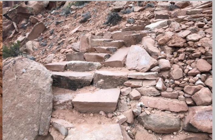
After – Retained slope with hardened surface trail
