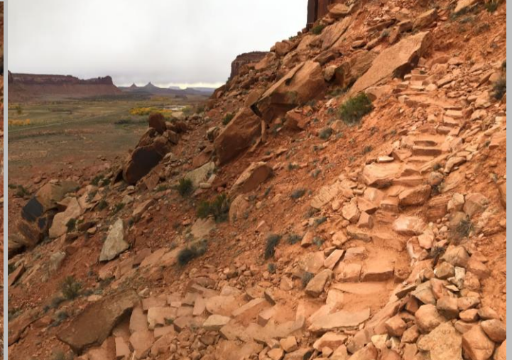
After – Stone structure constructed to provide a durable walking surface.
