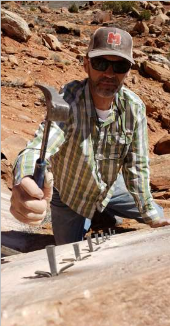
Stone Quarrying – 273 3ft of stone was quarried on site
